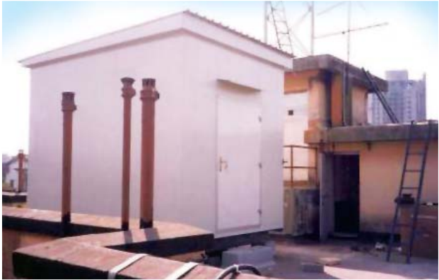
Shelters for Telecommunication & Transmission Systems all over India.
