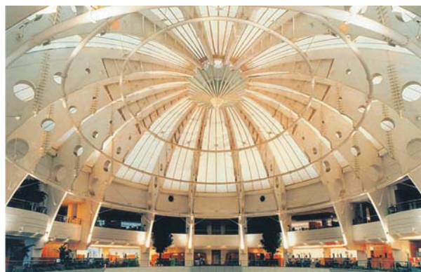
Structural Fire Proofing with Intumescent paint (2 hours fire rating) for ILFS building at Bandra Kurla Complex.
