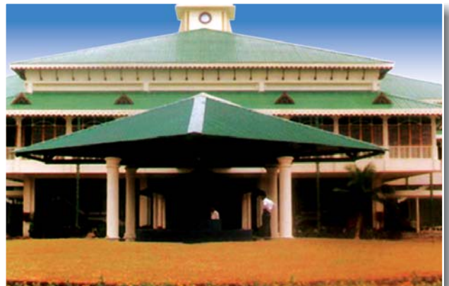
Lloydtile roofing at Galfar India Ltd., Convention Hall at Cochin.
