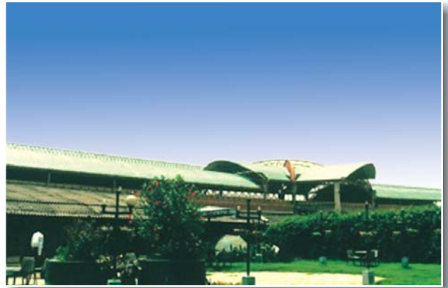
Roofing System for Delhi Metro Railway station.
