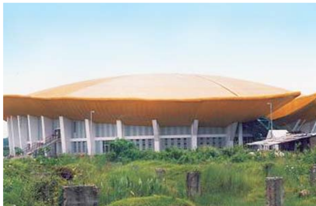
Roofing System at Rajeev Gandhi Stadium, Guwahati.
