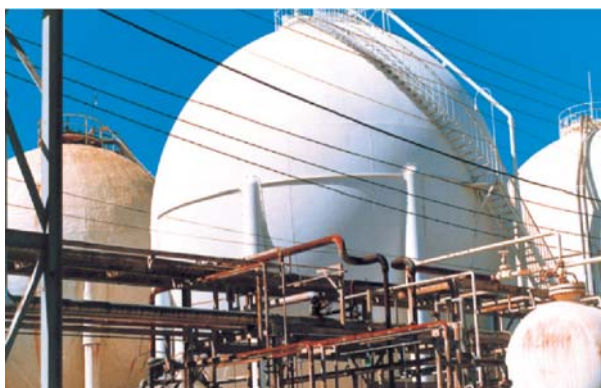
Thermal Insulation and fire proofing for low temperature storage spheres / tanks A/c. Various Petrochemical, Chemical & Fertiliser complexes all over India.
