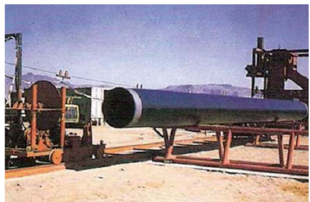
Coating & Wrapping at Reliance Industries Ltd., Jamnagar
