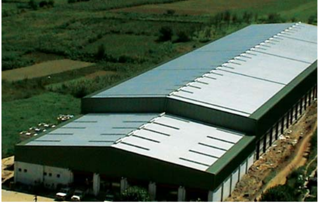
Pre-engineered structure with Gas tight Controlled Atmosphere Mega Cold Store Adani Agrifresh Ltd. Sanij, Himachal Pradesh.
