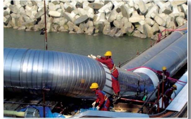
Cryogenic Insulation of Liquefied Natural Gas unloading pipelines for Shell LNG Terminal, Hazira. Operating Temperature of this Line is -165^{\circ}\text{C} . Total Insulated (finished) Area: 28000\text{m}^2 . Value of Contract: Rs. 14 Crores.
