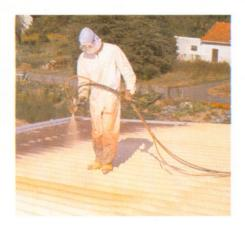
The SEAMLESS and MONOLITHIC nature of the sprayed foam provides a full proof method of sealing cracks and rendering any surface moisture resistance and draught proof. The closed cell foam has a low water vapour transmission properties and also inhibits ingress of moisture.
