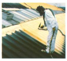
Although the foam forms a weather resistance membrane, a final coating is required as an additional protection against U.V. radiation in exterior applications. In the same way as any other organic material, polyurethane foam can eventually be attacked by the ultraviolet rays of the sun, hence a protective coating is necessary.
