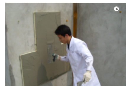
External Wall Insulation
