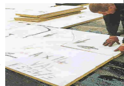
Roof Insulation - Overdeck
