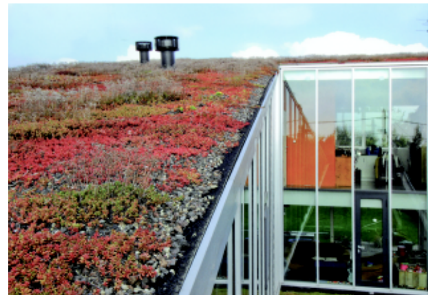
Roof Gardening over sprayed PUF Roof
